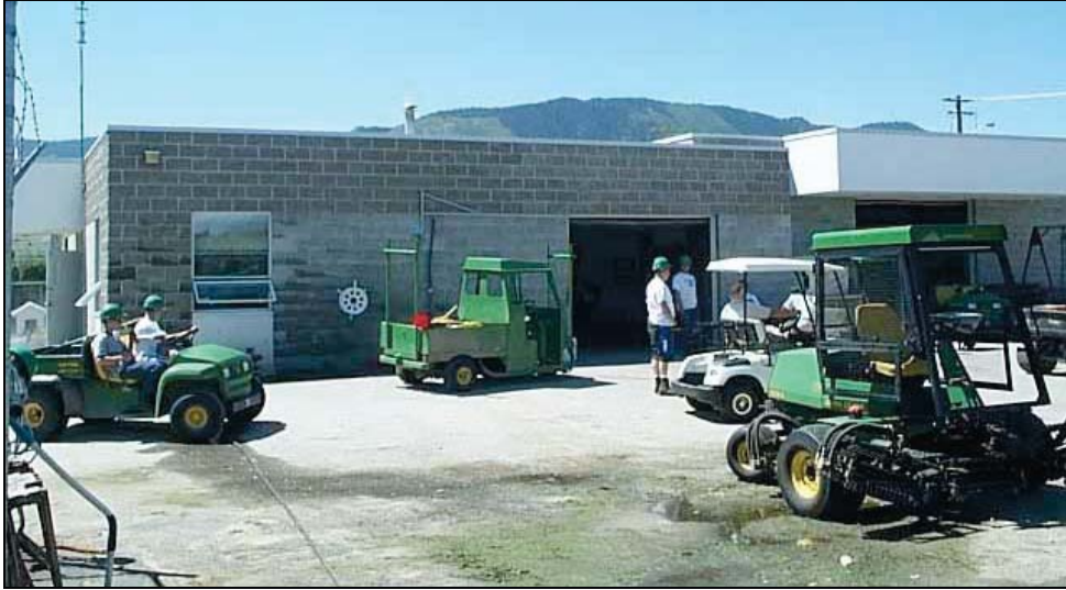
The Odyssey Maintenance Building
