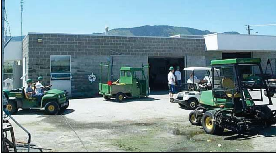
The Odyssey Maintenance Building
